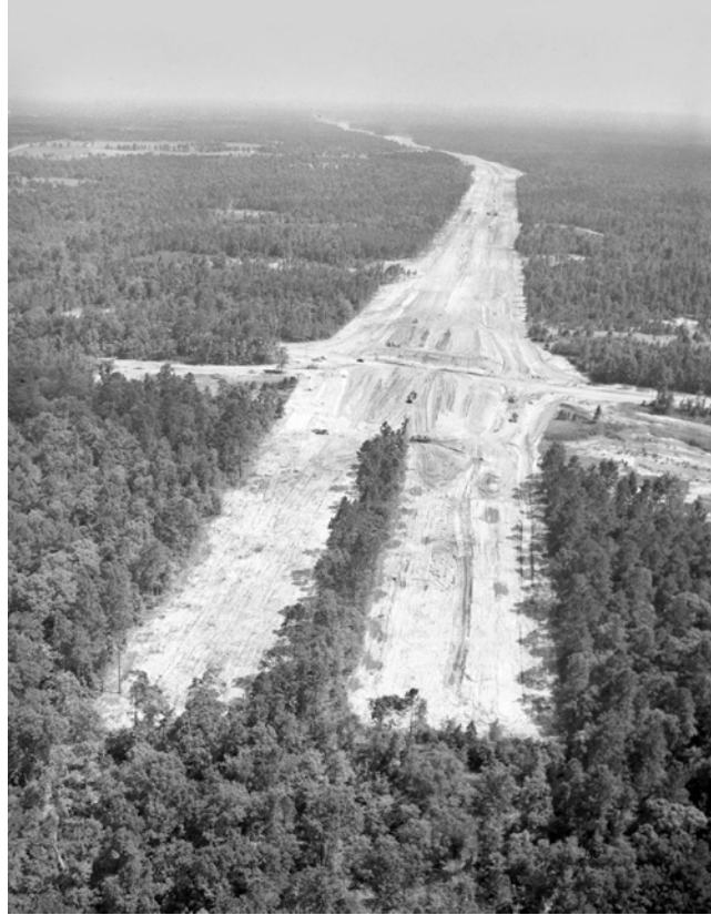
FIGURE 1.2 Early construction of Interstate 45 (I-45), Conroe, Texas. (© TxDOT.)
