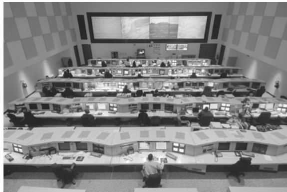
FIGURE 1.8 Houston TranStar control room. (© TxDOT.)
