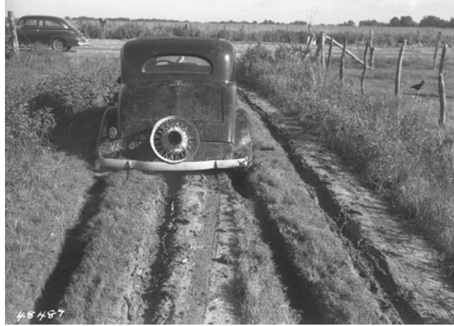
FIGURE 1.1 Vehicle stuck on a muddy roadway. (© Texas Department of Transportation [TxDOT].)
