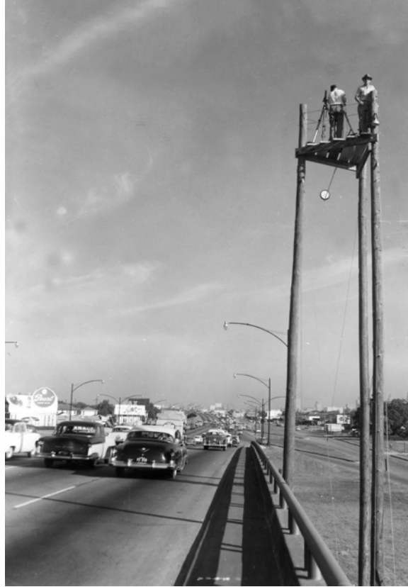
FIGURE 1.6 Early traffic monitoring on Interstate 45 (I-45) Gulf Freeway, Houston, Texas. (© TTI.)
