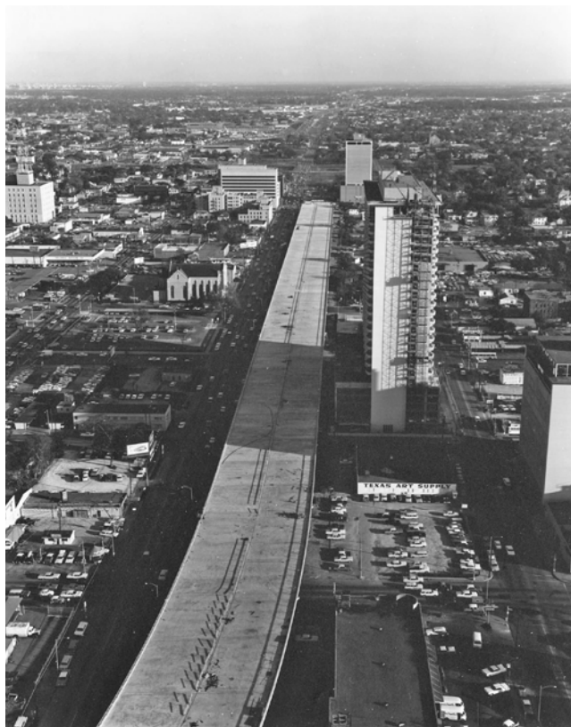
FIGURE 1.4 Construction of Interstate 45 (I-45) in Houston, Texas. (© TxDOT.)
