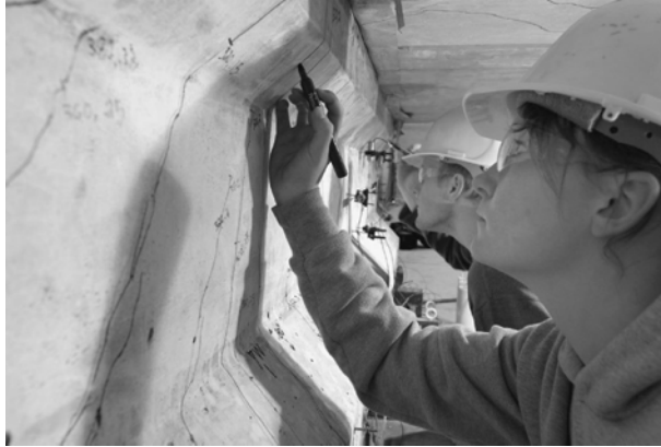
FIGURE 1.11 Bridge research and inspection. (© TTI.)
