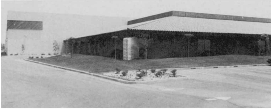
FIGURE 1.2A Foreground: Office portion of wood-frame construction. Background: Warehouse with concrete tilt-up walls and wood roof system. (Photo courtesy of Mike Hausmann.)
