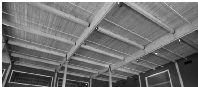
FIGURE 1.3 Interior of a building with a panelized roof system. (Photo courtesy of Southern Pine Council.)
